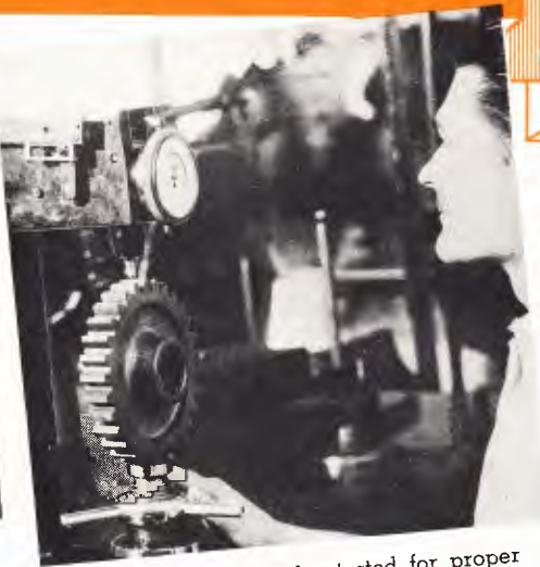
Finished gears are also tested for proper hardness on this Rockwell testing equipment. Properly hardened gears assure long gear life, freedom from break-downs in tractor operations.
